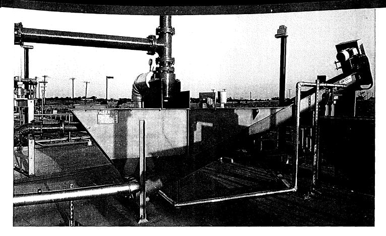
The dewatering **PISTA**<sup>®</sup> Grit Screw Conveyor is designed to work in concert with the complete **PISTA**<sup>®</sup> Grit Removal System, providing superb dewatering and high retention of fine grit without the burden of high maintenance. The **PISTA**<sup>®</sup> Grit Screw Conveyor boasts a sleek, compact design with a similar sleek footprint to S&L's **PISTA**<sup>®</sup> product line.
